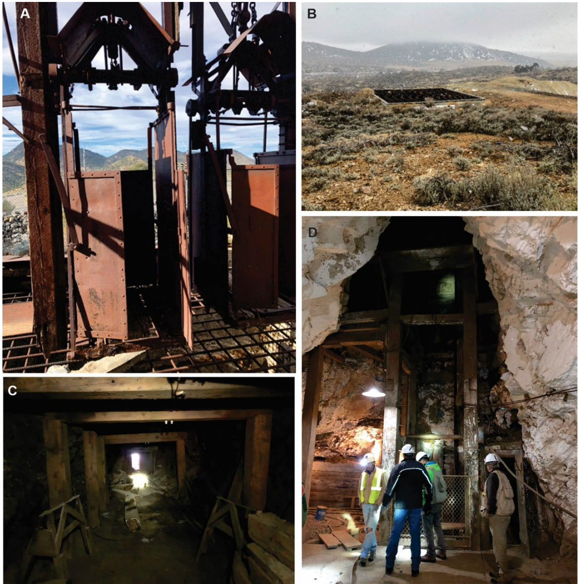
Figure 5-7: Examples of Underground Historical Infrastructure at the Tintic Project: (A) Grand Central Shaft; (B) Sunbeam Shaft Collar; (C) Mammoth Mine; and (D) Mammoth Mine Shaft Station at 300 Level Underground
